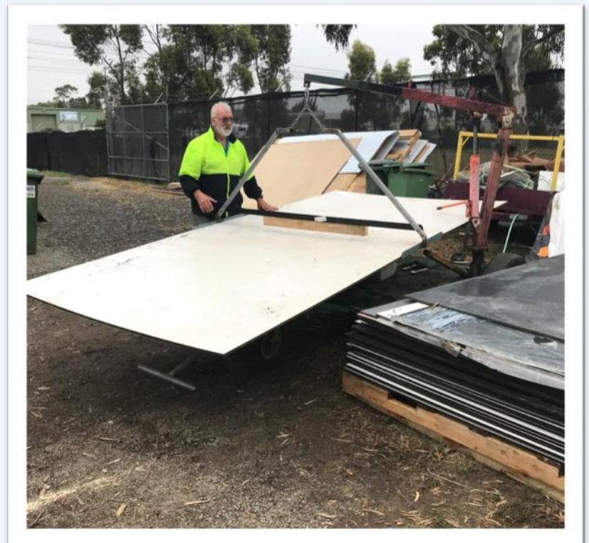
Kevin's latest back saving invention to handle our new Shed sheets of wall cladding donated by Laminex Industries .
