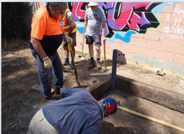
A bit of back breaking and surveying work
